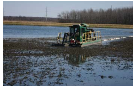
Pond Cleaning utilizing PMI's Industrial Dredge
