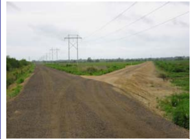
Landfill road construction
