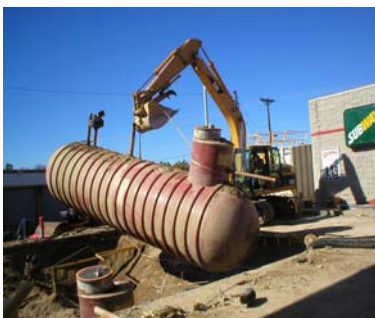
UST remediation & closure project.
