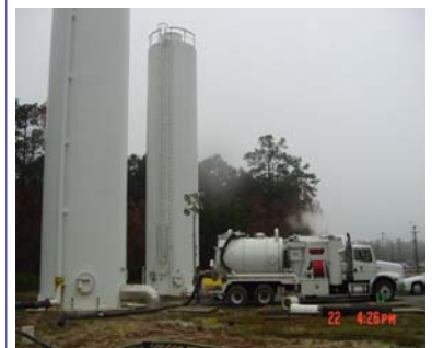
Vacuum Truck services to remove solids from water storage tanks.
