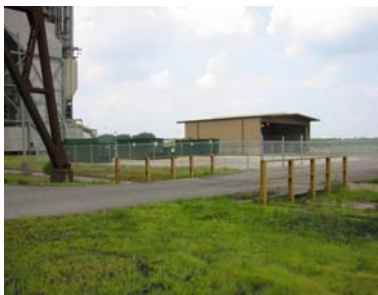
Solid waste collection facility
